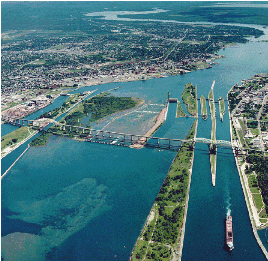
Aerial View of the Soo Locks on the St. Mary's River. Canada, to the left, the U.S. to the right.
