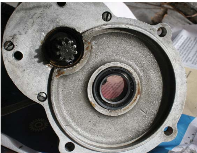
Photo 4 -New lower seal is in place
