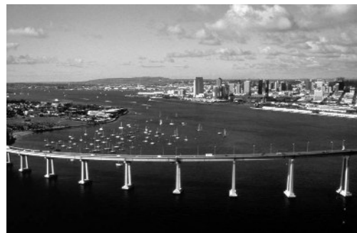
Coronado Bridge connecting San Diego and Coronado, California. Construction on the 2.1 mile bridge began in 1967. The span reaches 200 feet which allows U.S. Navy ships from the nearby San Diego Naval Station to pass underneath it.
