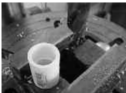
Ordinary butt-splice (note interior rib to be removed).
